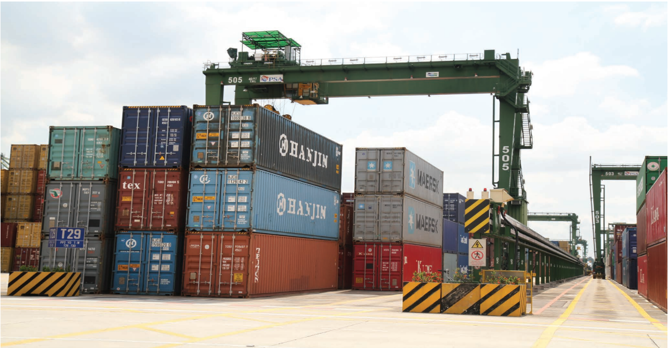
▲ Electric-automated RTG cranes at PPT. PSAC aims to progressively electrify all diesel-based port handling equipment and vehicles at its container terminals.
