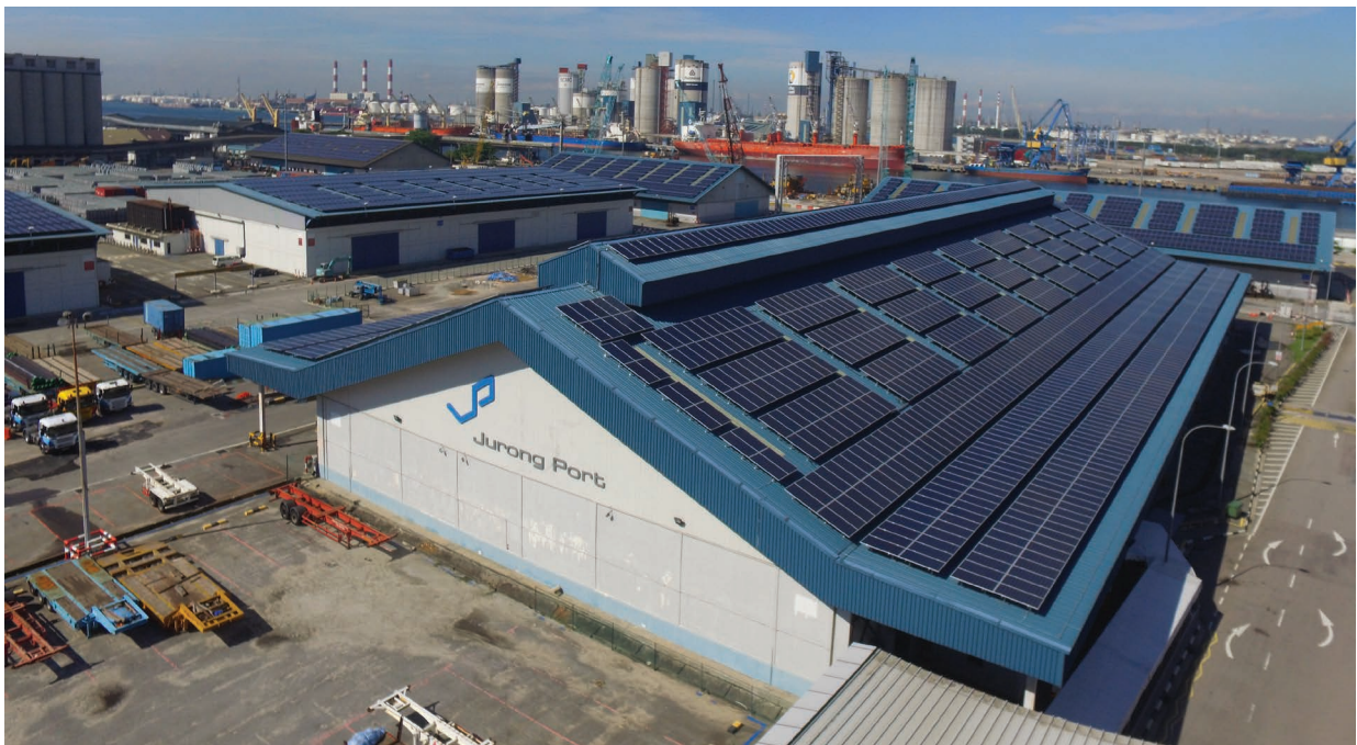
▲ Jurong Port's solar power generation facility offsets more than 10% of the port's electricity needs.
