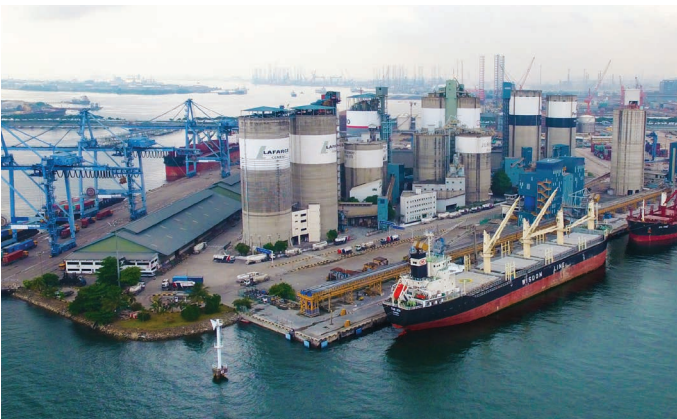
◀ Jurong Port has been the main gateway for general and bulk cargo into Singapore for more than 50 years. It is moving towards being a next generation multipurpose port by harnessing digitalisation and sustainability models that support the port's growth.
